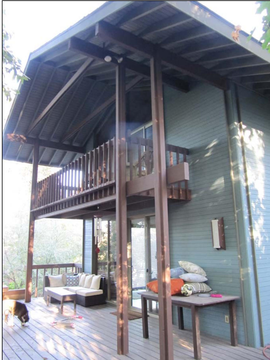
North elevation of Trogdon House in 2016, looking east
