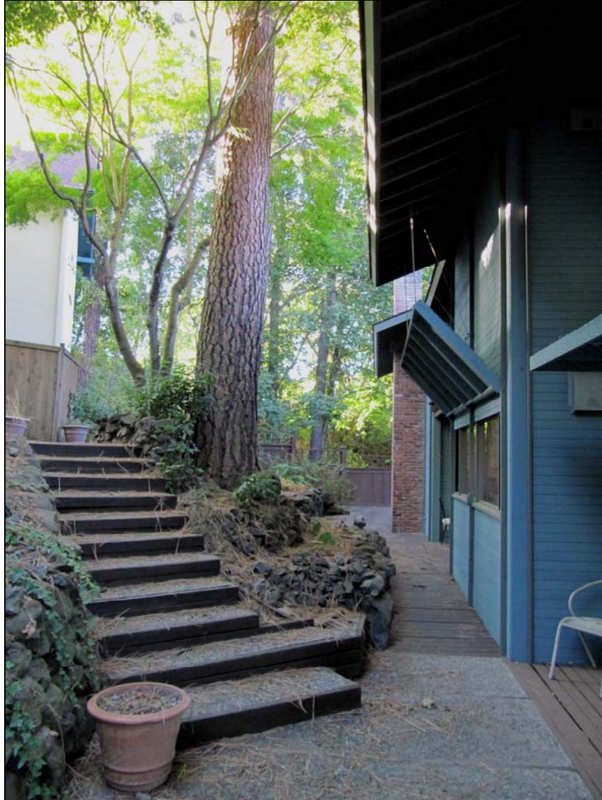
West rear elevation of Trogdon House in 2016, looking north
