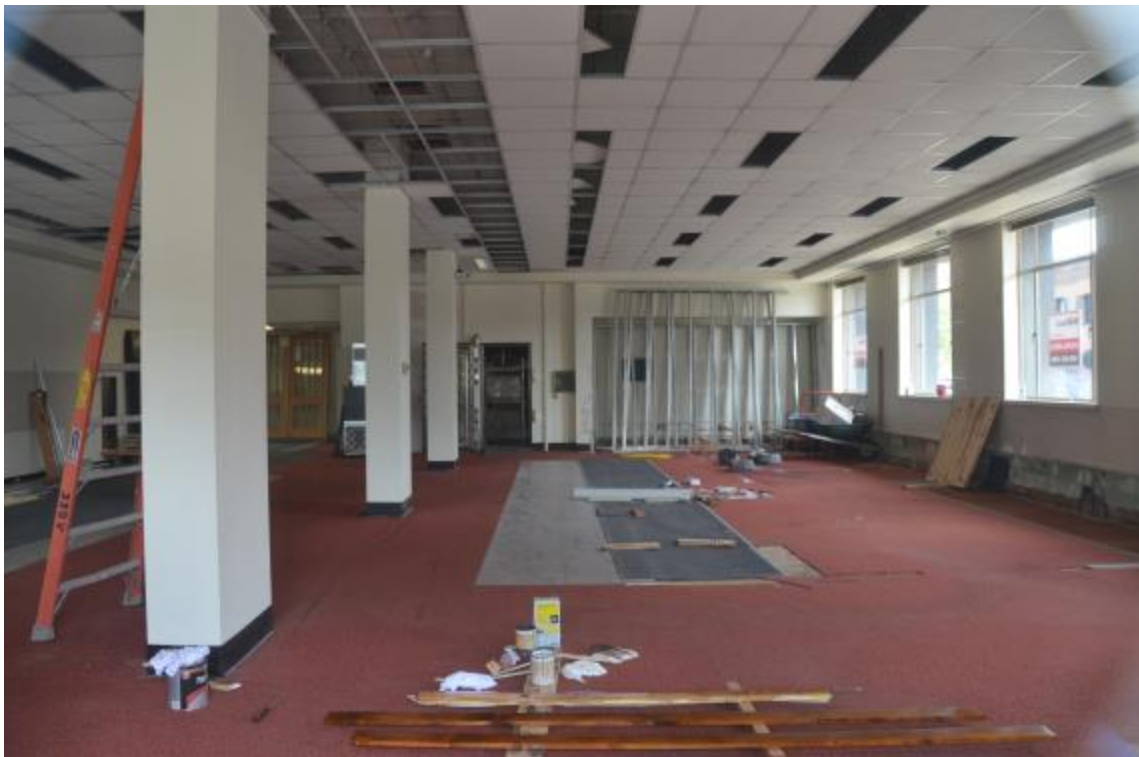
19. Interior View of former SeaFirst Bank, Bays 1 & 2, looking east
