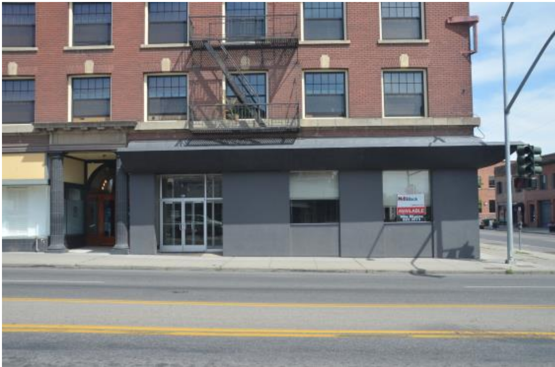
9. First floor retail bays 1 & 2 and main entry, looking east
