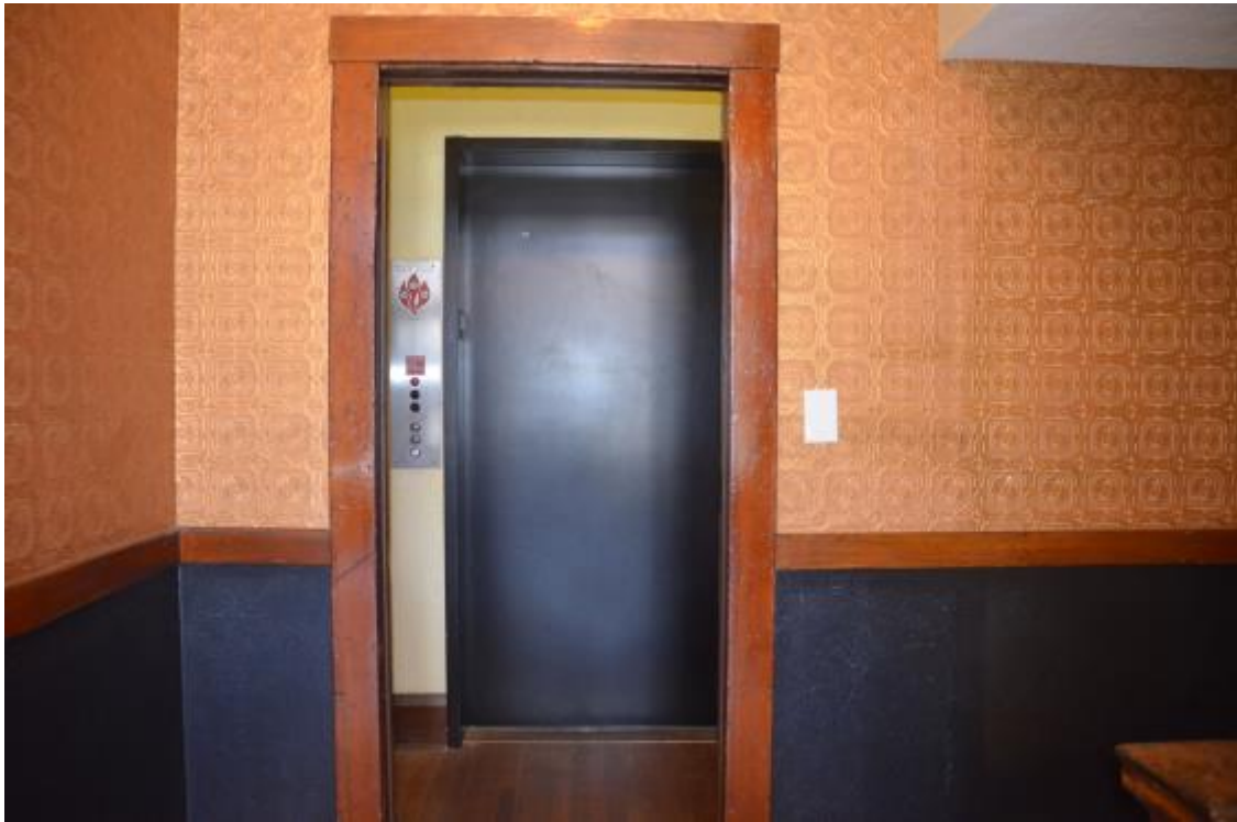
22. First floor lobby - elevator alcove
