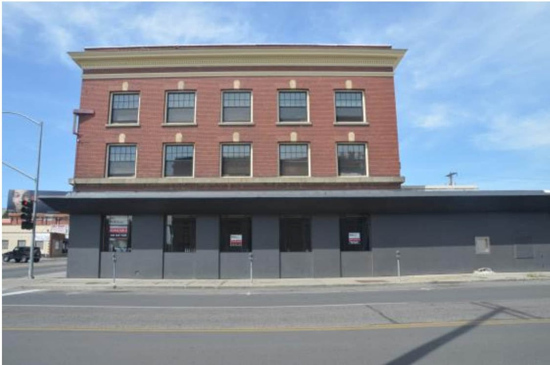
5. South facade, view to the north
