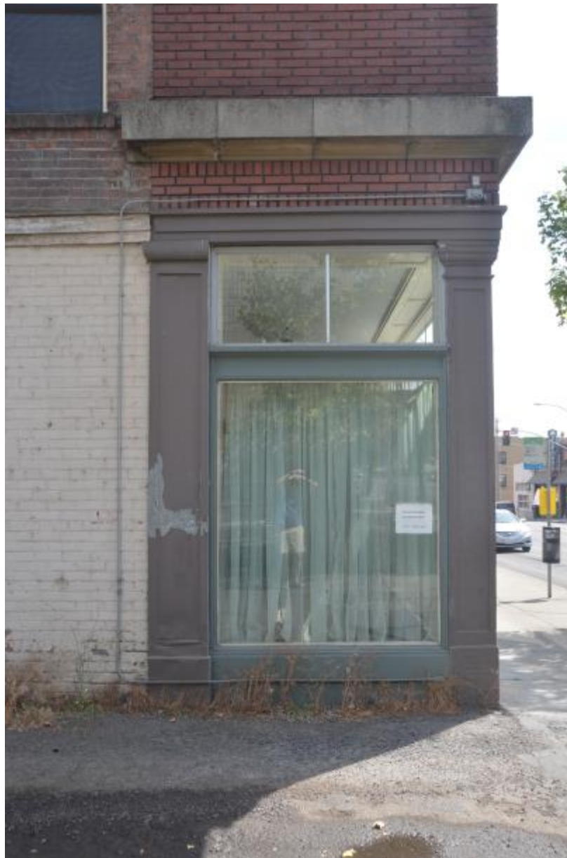
12. Northwest corner, north facade, looking south
