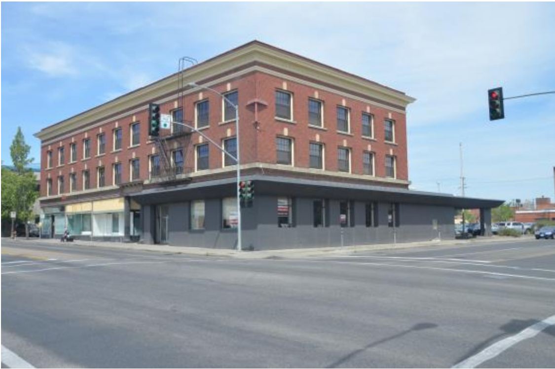
3. SW corner of building, west and south facades, view to the NE
