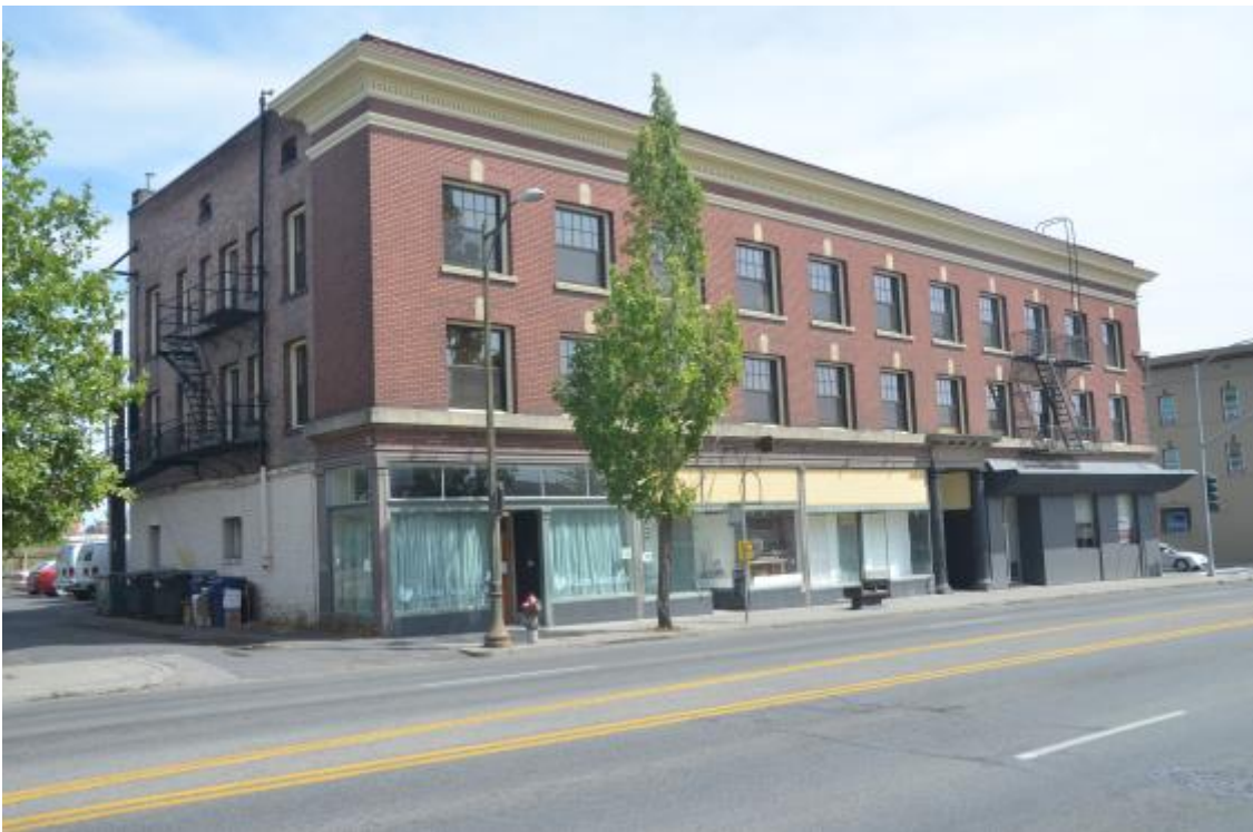
4. NE corner of building, north and west facades, view to the SE
