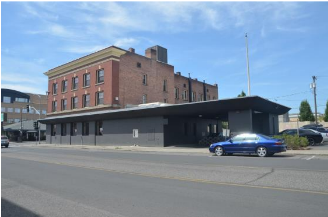
6. SE corner of building, south & east facades, view to the NW
