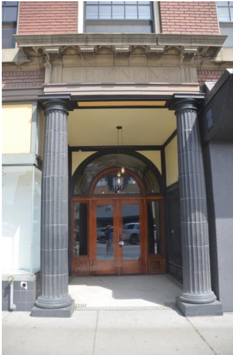
10. Main entry portico & alcove, looking east
