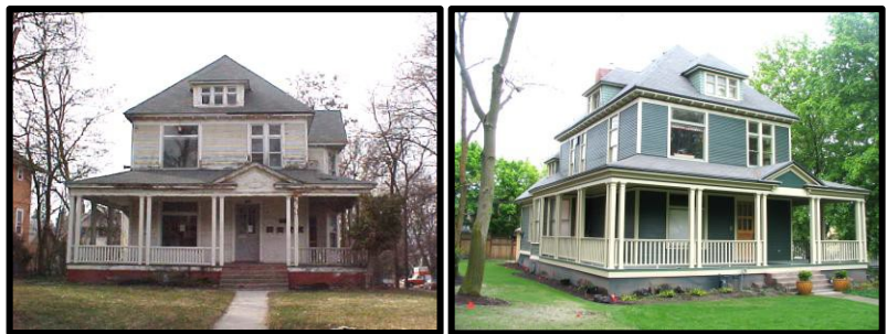
Thomas J. Graham House before and after rehabilitation.
